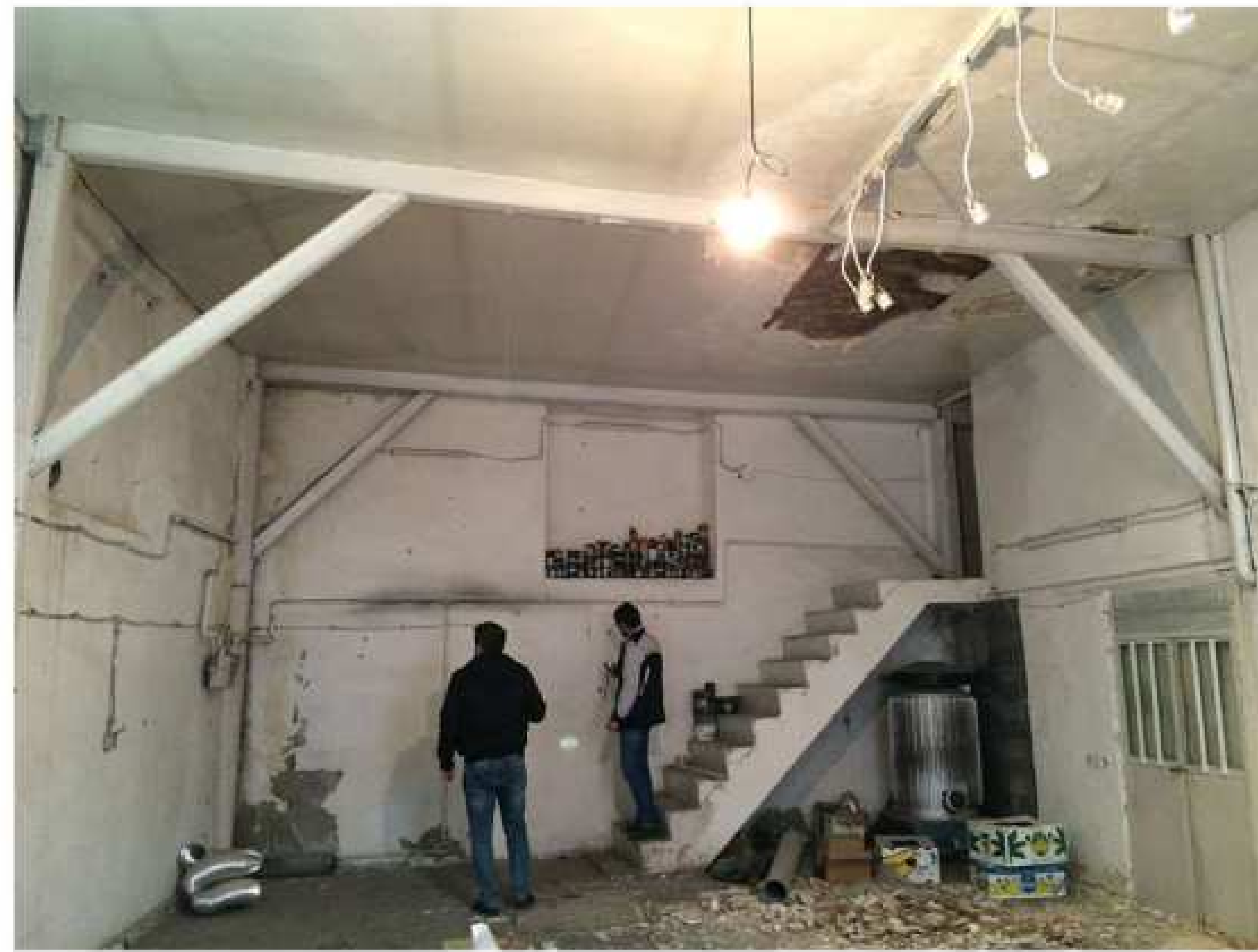
EXISTING INTERIOR ELEVATION
