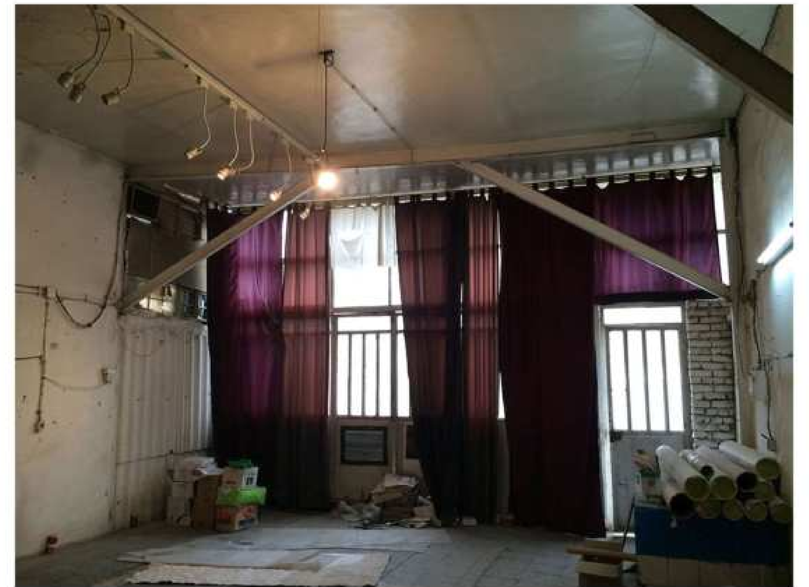
EXISTING INTERIOR ELEVATION
