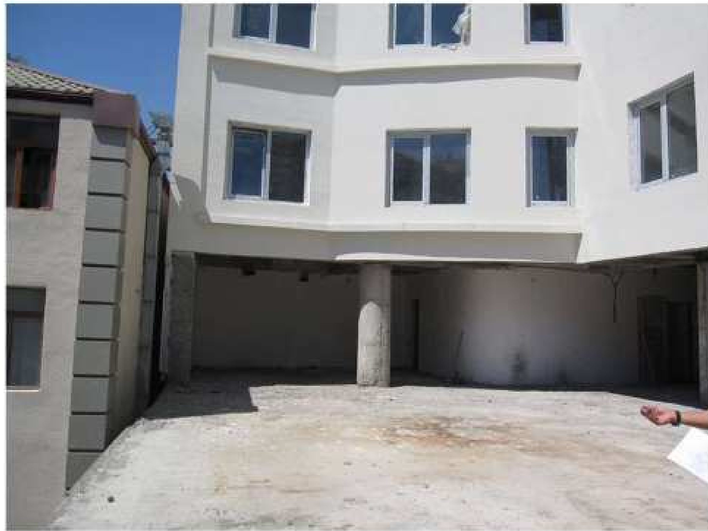
Existing Space - Second Floor
